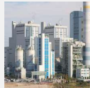
10MW plant completed
