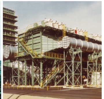
• Wet Type Horizontal Flow ESP
