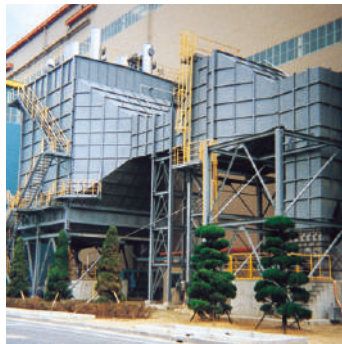
• Wet Type Vertical Flow ESP
