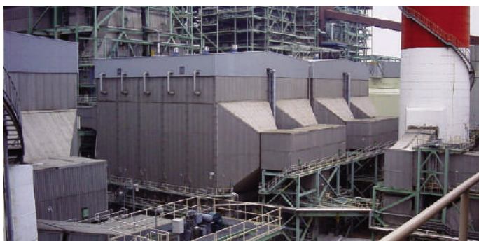
• Boryeong Thermal Power Plant Units 1~8
